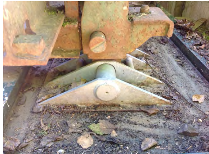
end post bearing - typical
