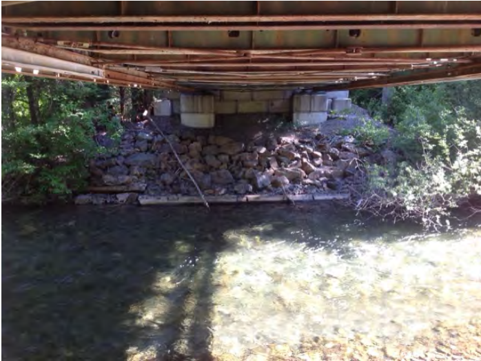
Right Bank Abutment when facing downstream
