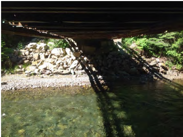
Left Bank Abutment when facing downstream
